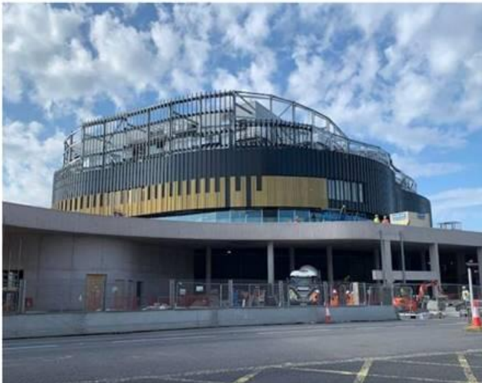
Arena – cladding / LED's being installed
